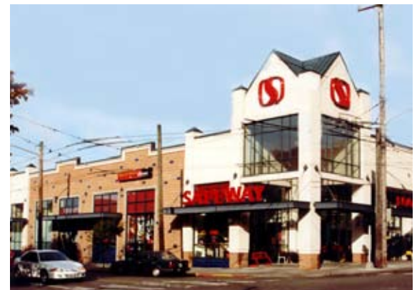
This grocery store is a good example of a well-designed corner entrance.
