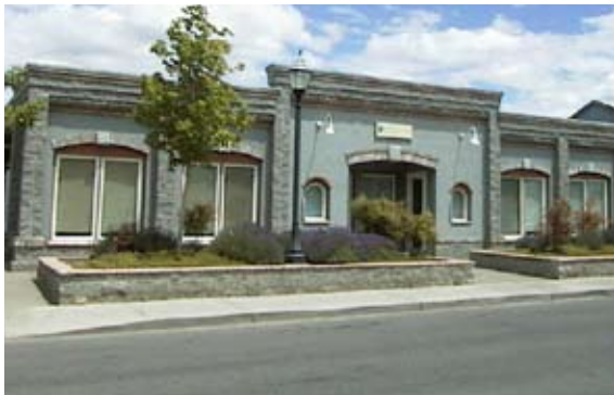
This commercial building utilizes concrete brick to create an aesthetically pleasing design.
