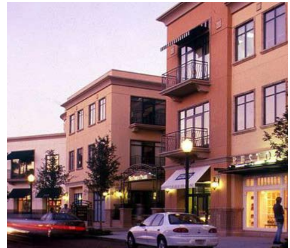
This is an example of a neighborhood street in a Town Center.
